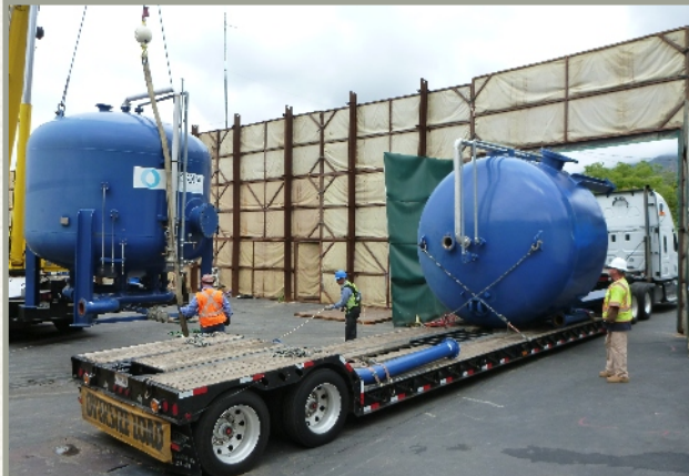
The temporary treatment system is removed
