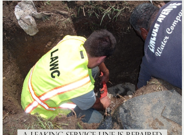
A LEAKING SERVICE LINE IS REPAIRED
