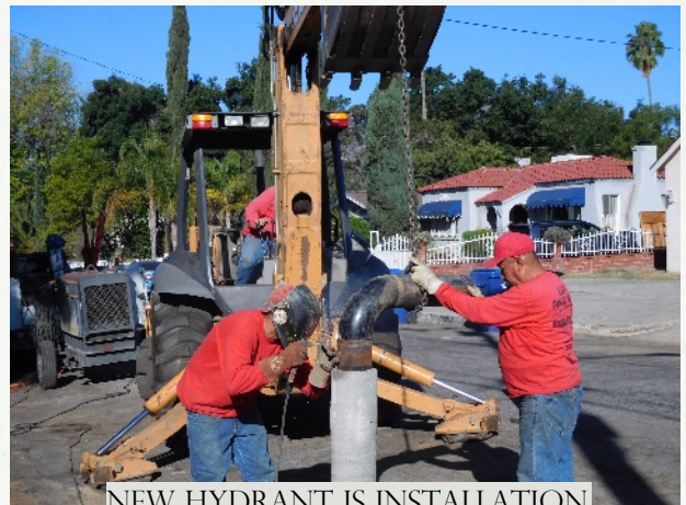
NEW HYDRANT IS INSTALLATION ON W MARIPOSA
