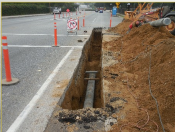
A joint is sealed with concrete
