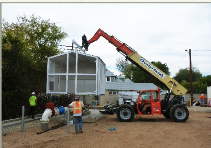
The well housing is delivered and assembled
