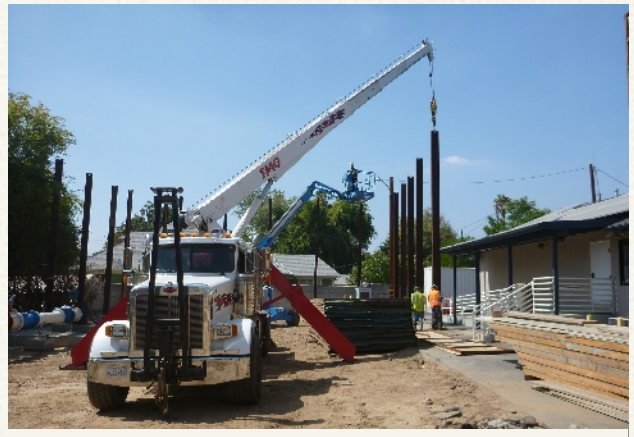
The sound wall structure is dismantled.
