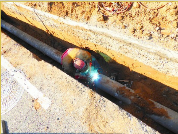
Sections of pipe welded together
