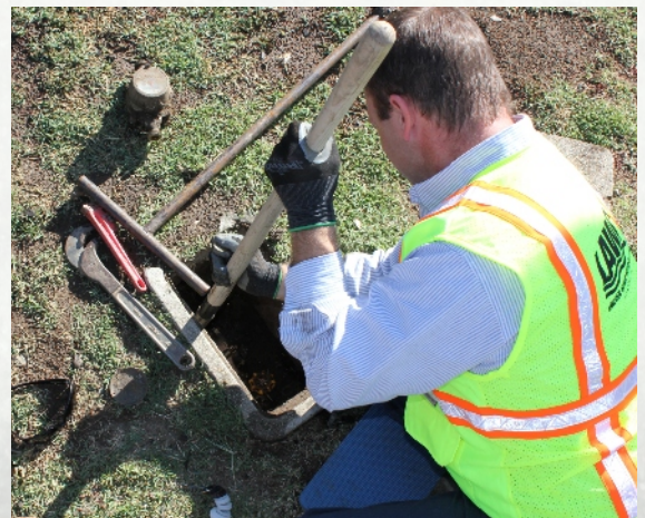
A NEW METER IS INSTALLED ON DEVIRIAN
