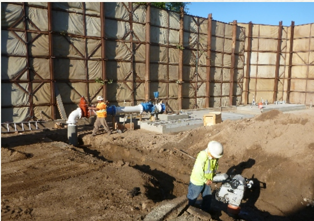
The effluent pipe and pump line are installed
