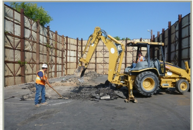
Asphalt is removed to begin grading
