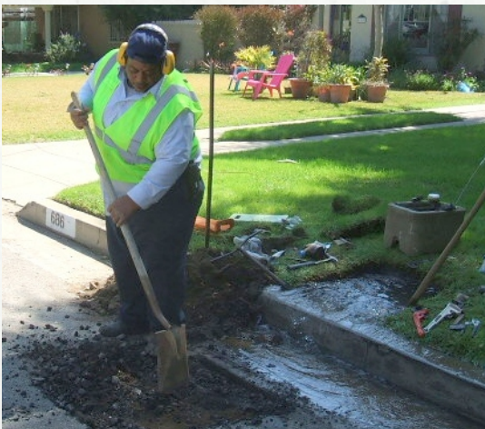
THE ROAD IS CUT AND EXCAVATED TO REPAIR A LEAKING SERVICE LINE
