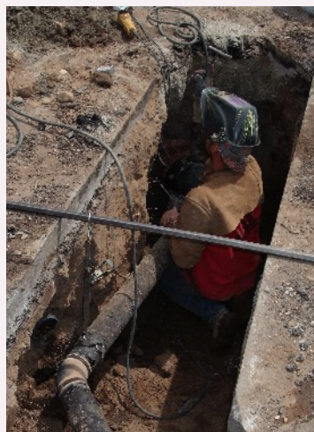
Old 4" pipe being removed.
