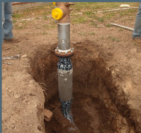
A new fire hydrant is installed.
