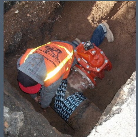
A valve is connected to the water main.
