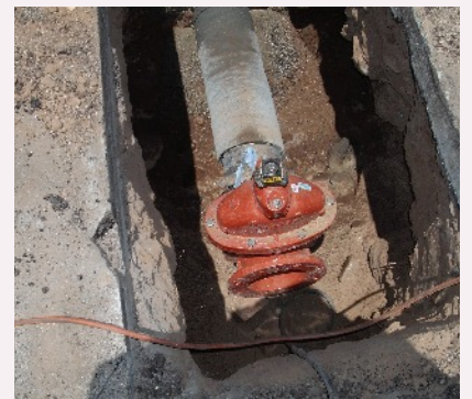
The water isolation valve is installed on the new pipe.
