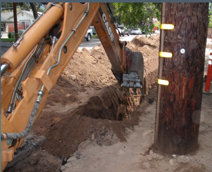
Trenching for the new pipeline.
