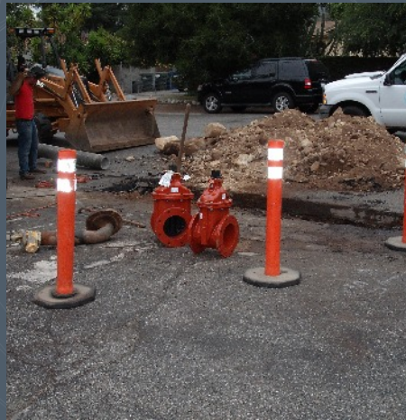
System isolation valves are ready to be installed.
