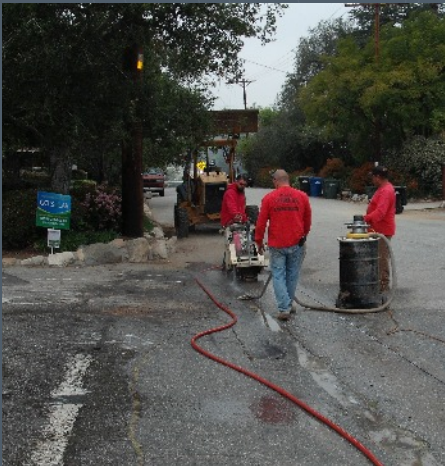
The pavement is marked and cut for trenching.
