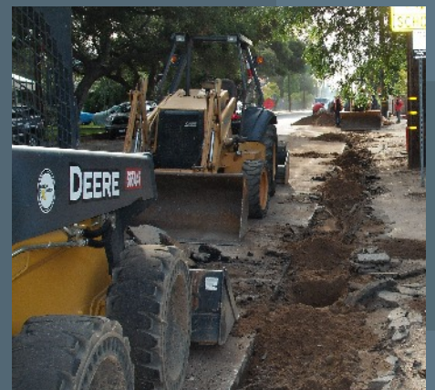
The trench is backfilled.
