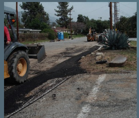
The ground is patched and prepared for the final paving.
