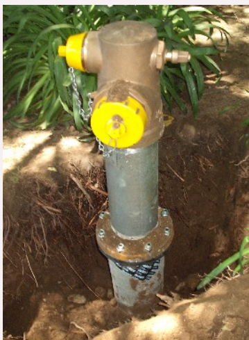
New hydrant is installed.
