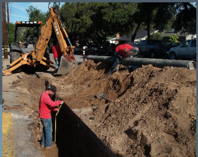
The depth of the trench is measured & inspected.
