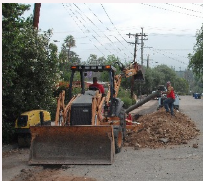
A section of pipe is guided into the ditch for installation.
