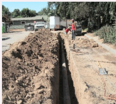
An extended view of the 20-foot section of new steel pipeline.
