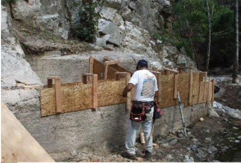
The catch box which was destroyed during the heavy rains and debris flow is repaired.
