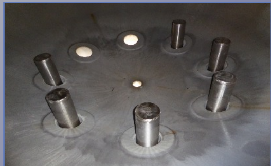
The stainless steel septa screens are an important part of the ion exchange vessel.
