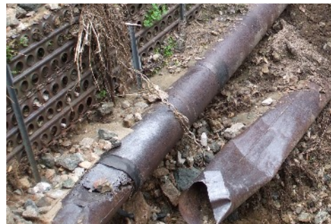
Several portions of the broken conveyance system were located on steep hillsides.
