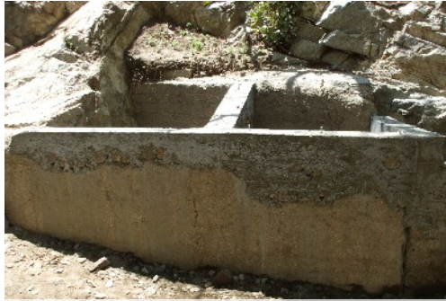
The catch box which was destroyed during the heavy rains and debris flow is repaired.
