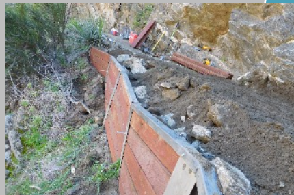
Retaining walls were constructed to stabilize the trail and reduce erosion.
