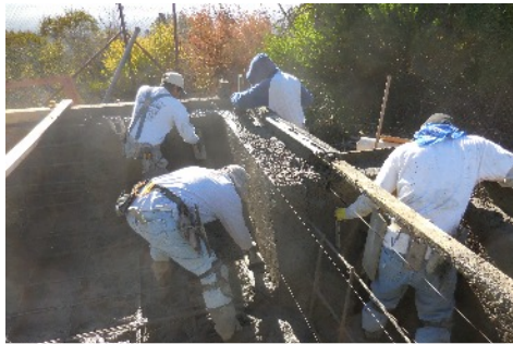
Concrete is applied to the wood frame.
