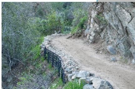
Retaining walls were constructed to stabilize the trail and reduce erosion.
