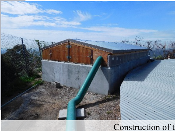
Canyon water is filtered then flows into the raw water reservoir.
