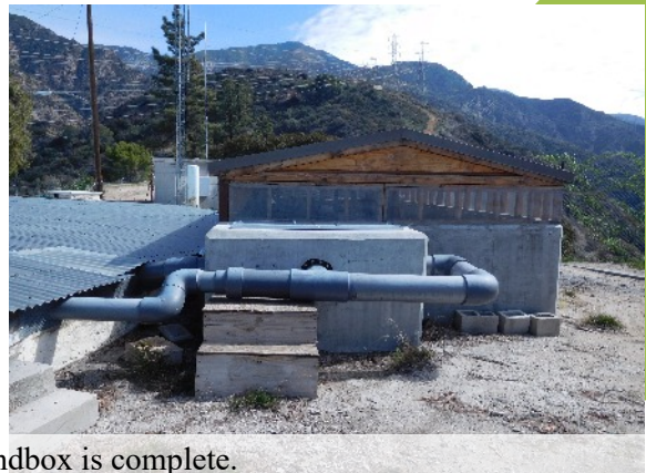
Canyon water is filtered then flows into the raw water reservoir.
