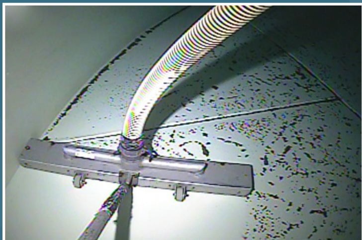
Sediment is removed from the reservoir floor.
