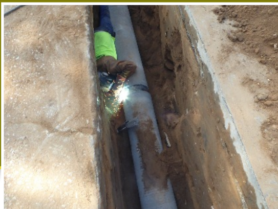
Two sections of pipe are welded together.
