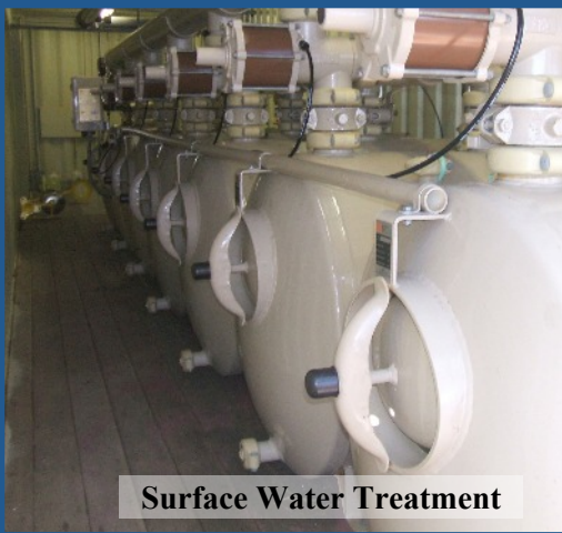
Granular Activated Carbon VOC Removal System
