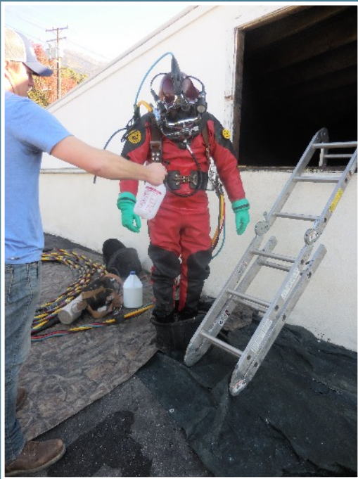
The diver is disinfected with liquid chlorine before entering the reservoir.
