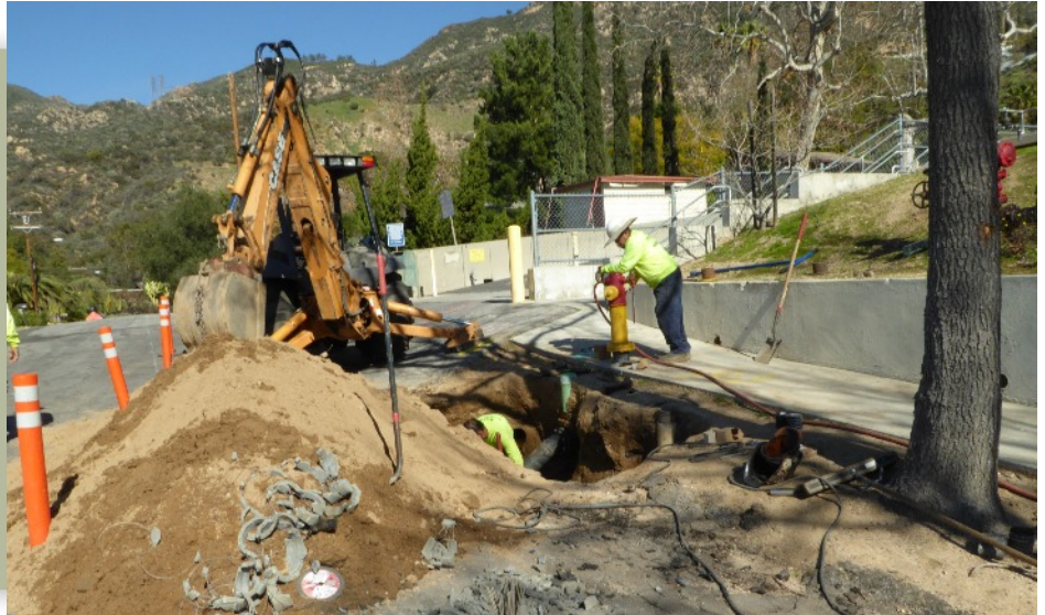
A new fire hydrant is installed.
