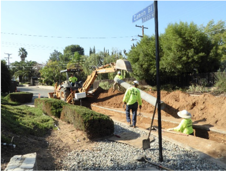
A 20-foot section of pipe is lowered into the trench.
