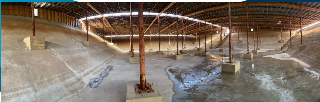
A panoramic view of the drained reservoir.
