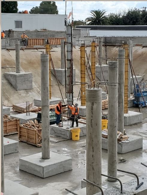
The column form is secured into place and prepped for concrete pour.
