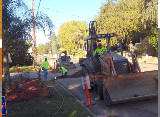
New service lines and meters are installed.
