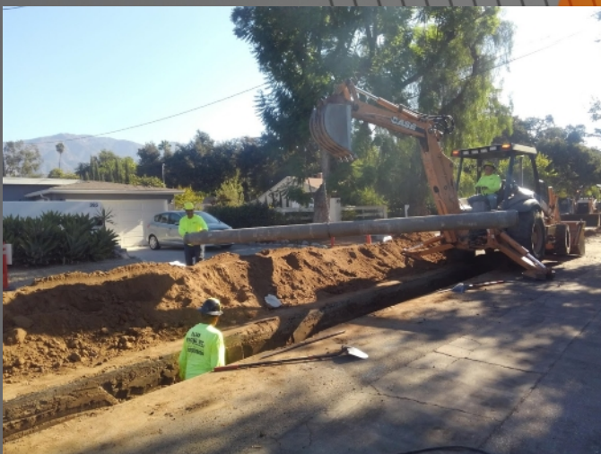
The pipe is lowered into place.
