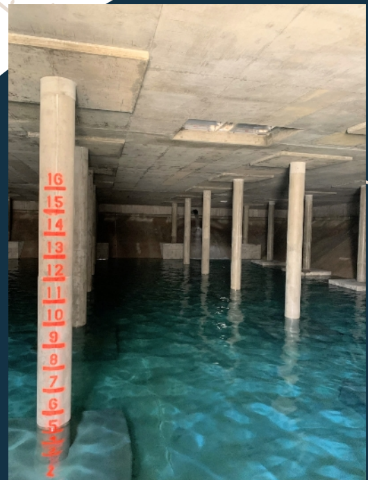
A view of the interior as the reservoir is refilled.
