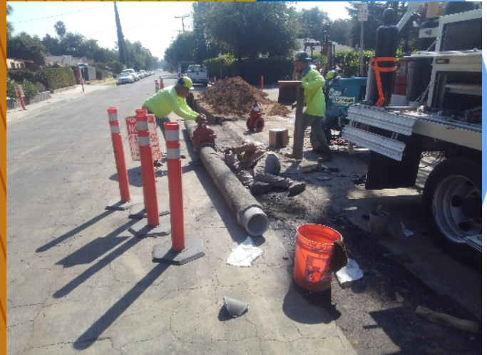
An isolation valve is installed on a section of pipe.
