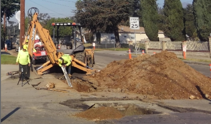
An adjacent water main connection is exposed and prepared to be connected to the new pipeline.
