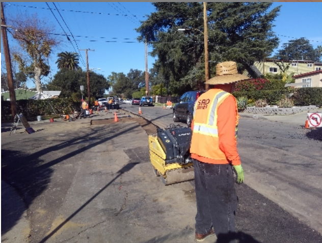
Final paving marks the completion of this project.
