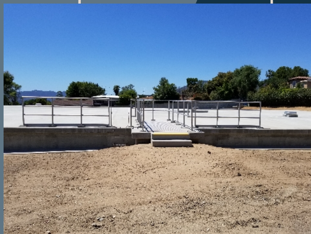
The new secured entrance into the reservoir.
