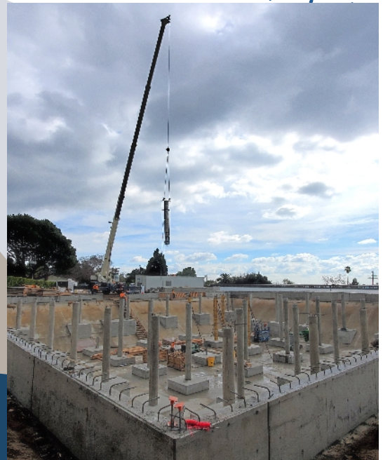
The column form is assembled, then the crane is used to lower it into the reservoir.
