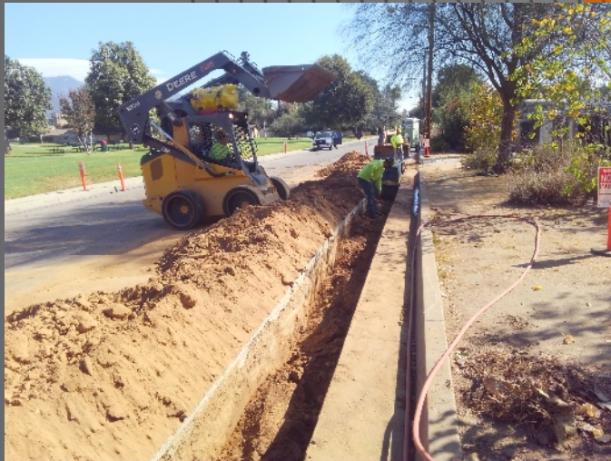
An adjacent water main connection is exposed and prepared to be connected to the new pipeline.
