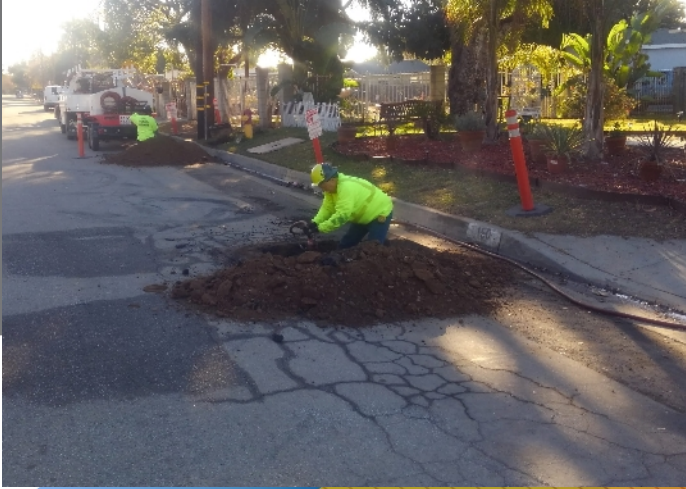
New service lines and meters are installed.
