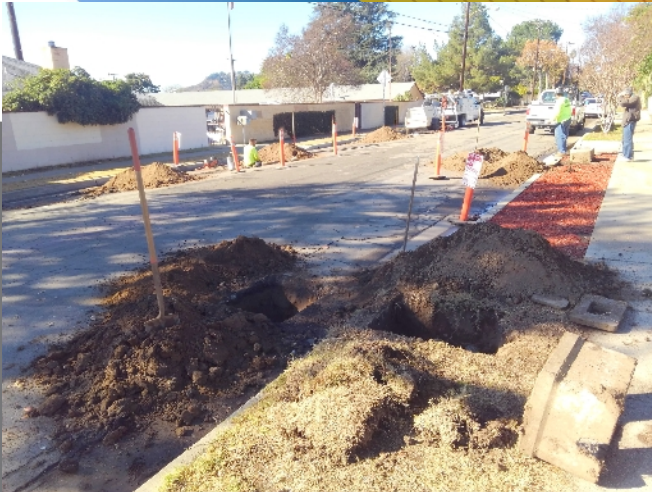
New service lines and meters are installed.
