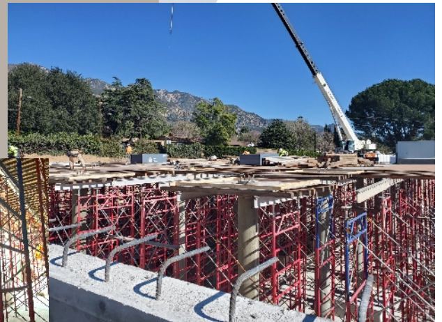
Following the completion of the columns, scaffolding is erected to support the form for the roof.
