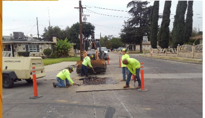
The ditch is covered with a metal plate and secured so traffic can safely resume.
