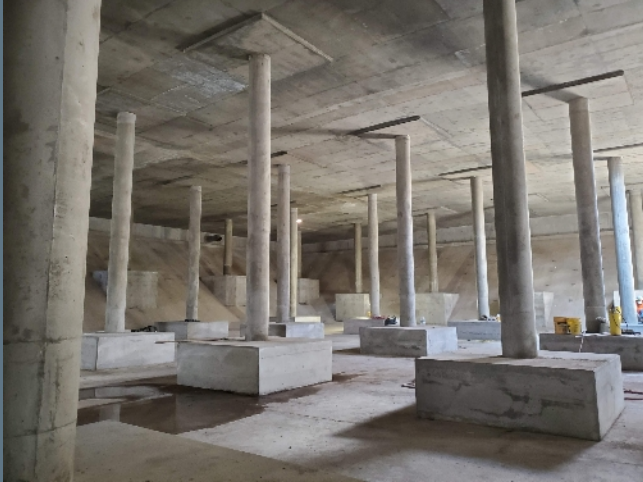
The reservoir interior.
