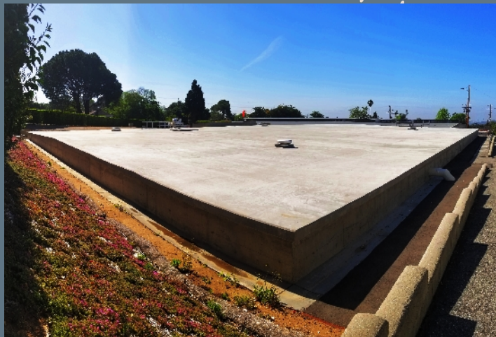
Northwest corner looking southeast.
