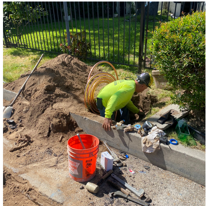
ONCE THE PIPE IS INSTALLED, THE TRENCH IS BACKFILLED AND COMPACTED.
