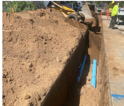
ONCE THE PIPE IS INSTALLED, THE TRENCH IS BACKFILLED AND COMPACTED.
