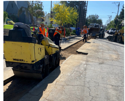
ONCE THE PIPE IS INSTALLED, THE TRENCH IS BACKFILLED AND COMPACTED.
