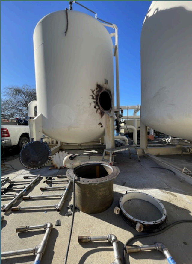
Justin La Point and Andres Estrada disassemble the interior laterals.
