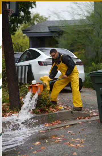
Andy Estrada tests the flow of a fire hydrant.
