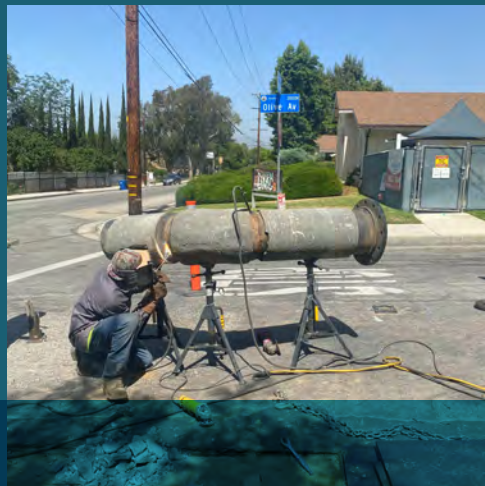
An adjacent pipeline is prepped to be tied into the new line.
