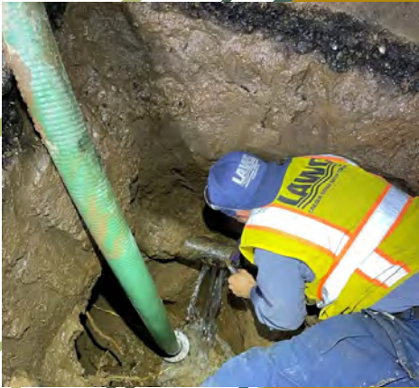
Andy Estrada prepares a leaking pipe to be clamped.
