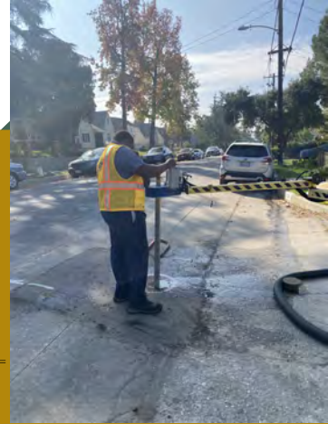
Jeremy Rogers shuts down a leaking street valve.
