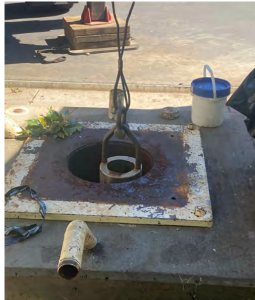
The careful process of extracting 800 feet of column pipe and the pump takes several hours to completed.
