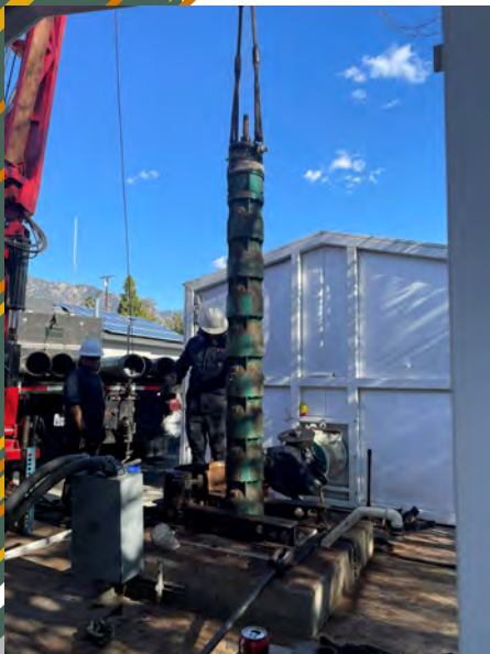
The careful process of extracting 800 feet of column pipe and the pump takes several hours to completed.
