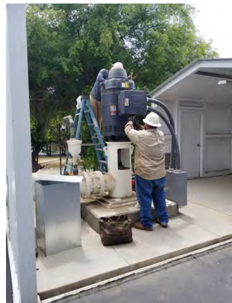
The motor is reinstalled and undergoing testing.
