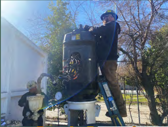
The 350 HP motor is disconnected and prepared for removal.
